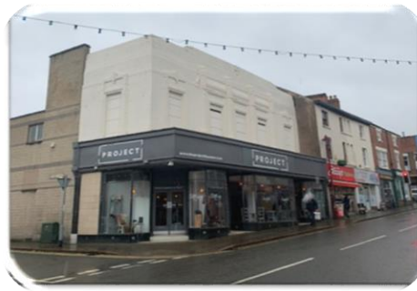
Former Woolworths Store, The Project, Bath Street, Ilkeston (ERE/0512/0002)
