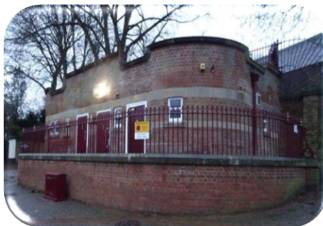
Public toilets, Market Place, Ilkeston (ERE/0512/0002)
