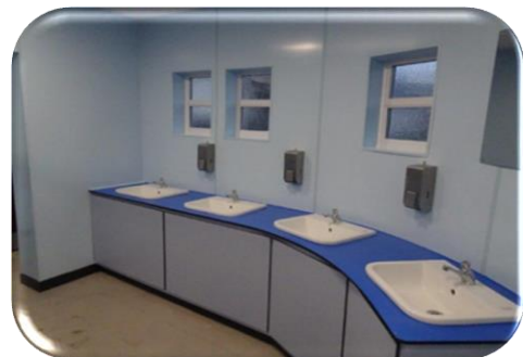
Public toilets, Market Place, Ilkeston (ERE/0512/0002)
