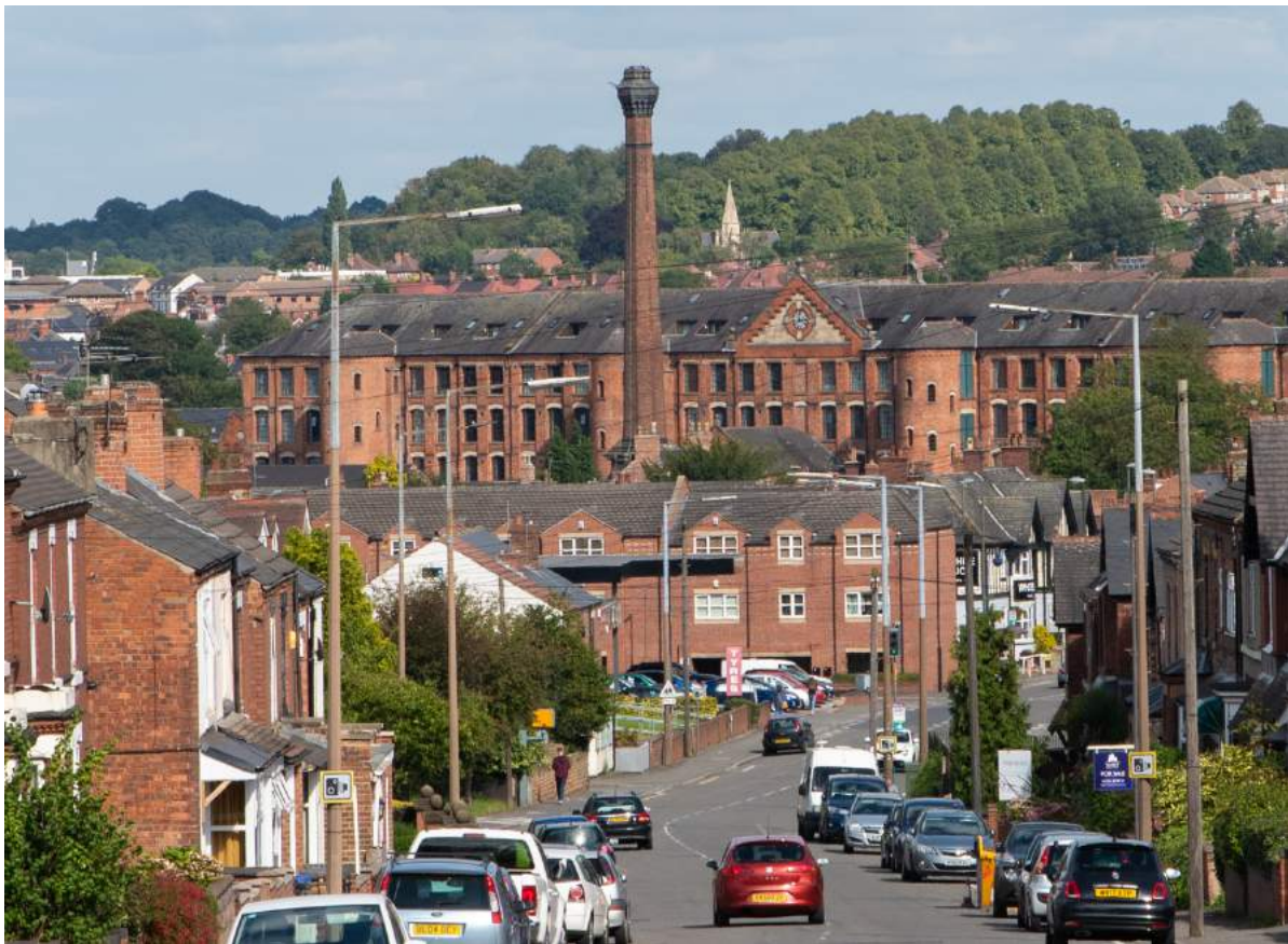
Long View down Derby Road towards Springfield Mill
