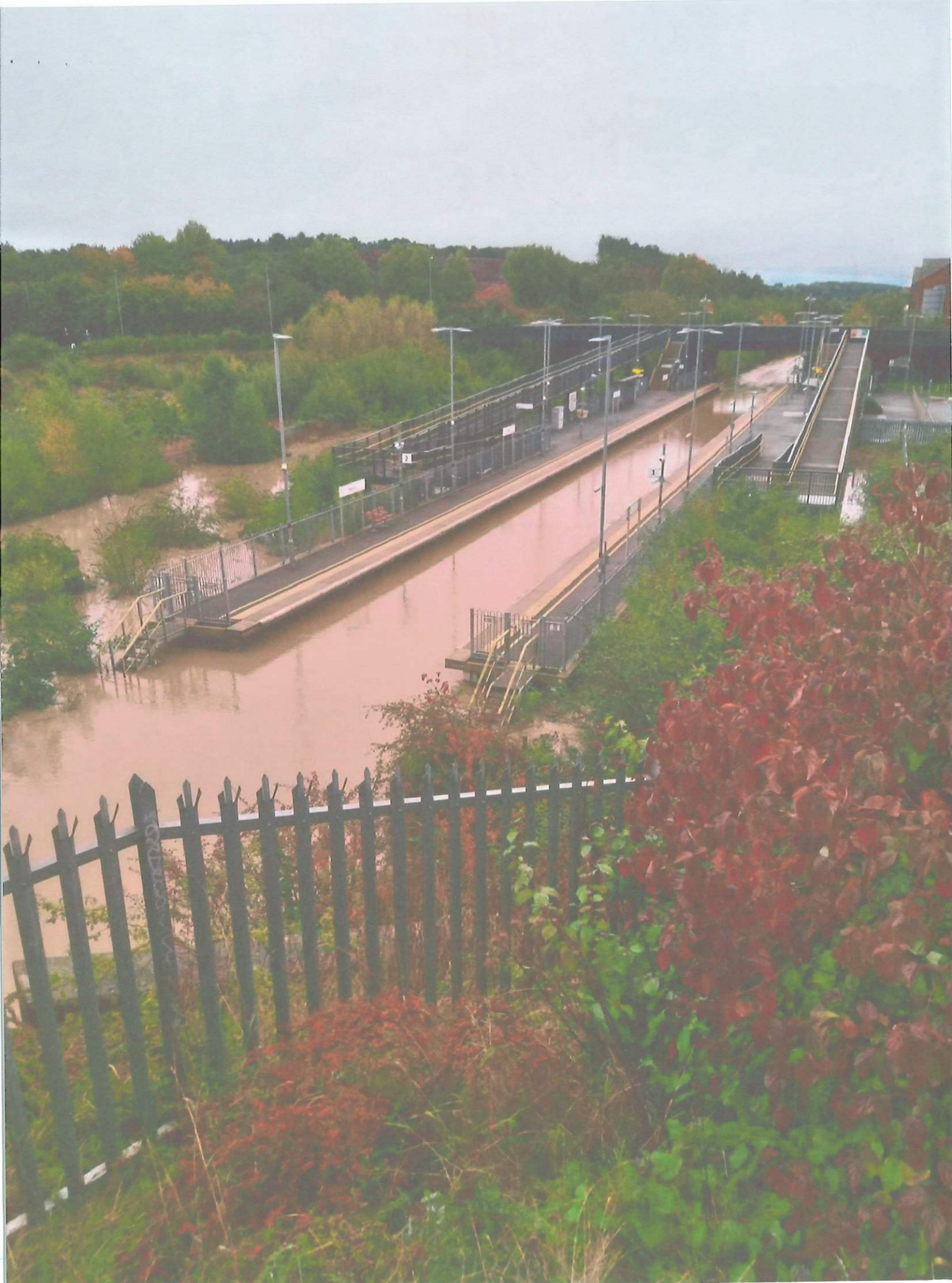
* I LIKESTON TRAIN STATION 20/10/23
